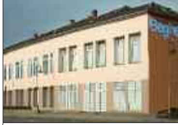
Beghelli Elplast Brno, Czech Republic
